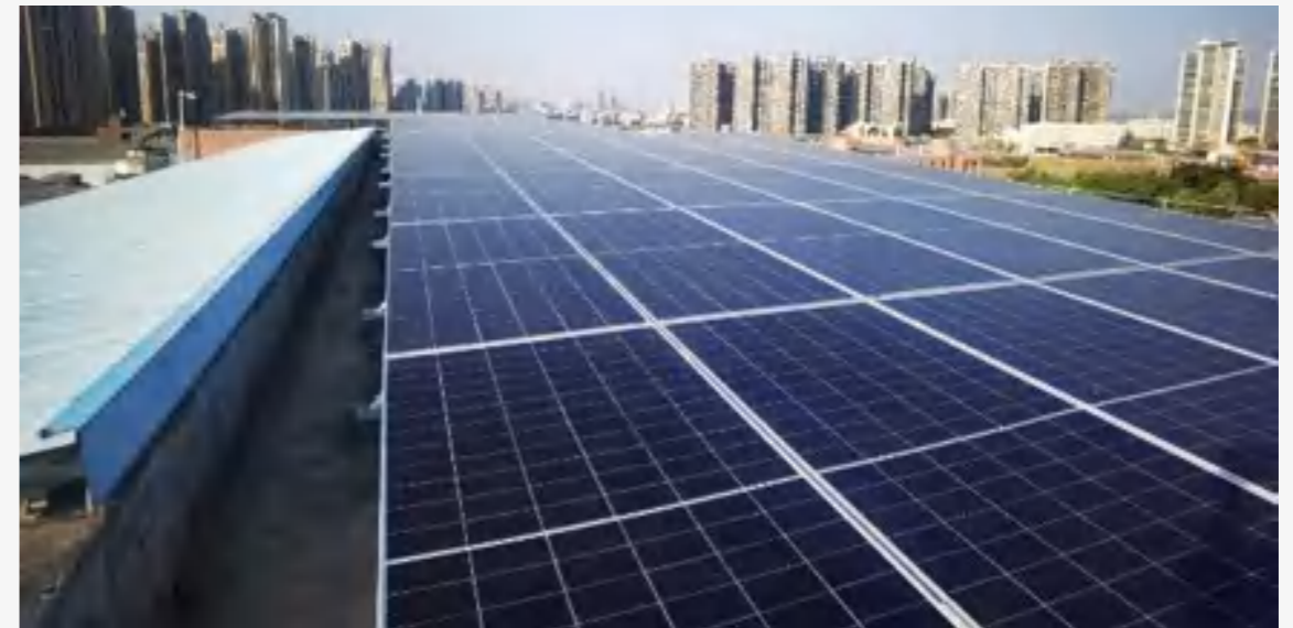
The Huizhou Highpower 0.88 MWp Photovoltaic Project was Successfully Completed and Commissioned in November 2025, Contributing to the Optimization of the Energy Structure
